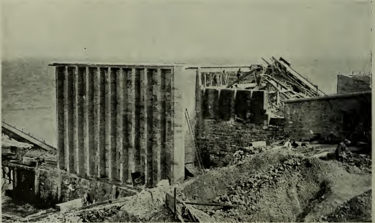
REINFORCED CONCRETE LIMESTONE BUNKER, CAPACITY 4,000 TONS.
